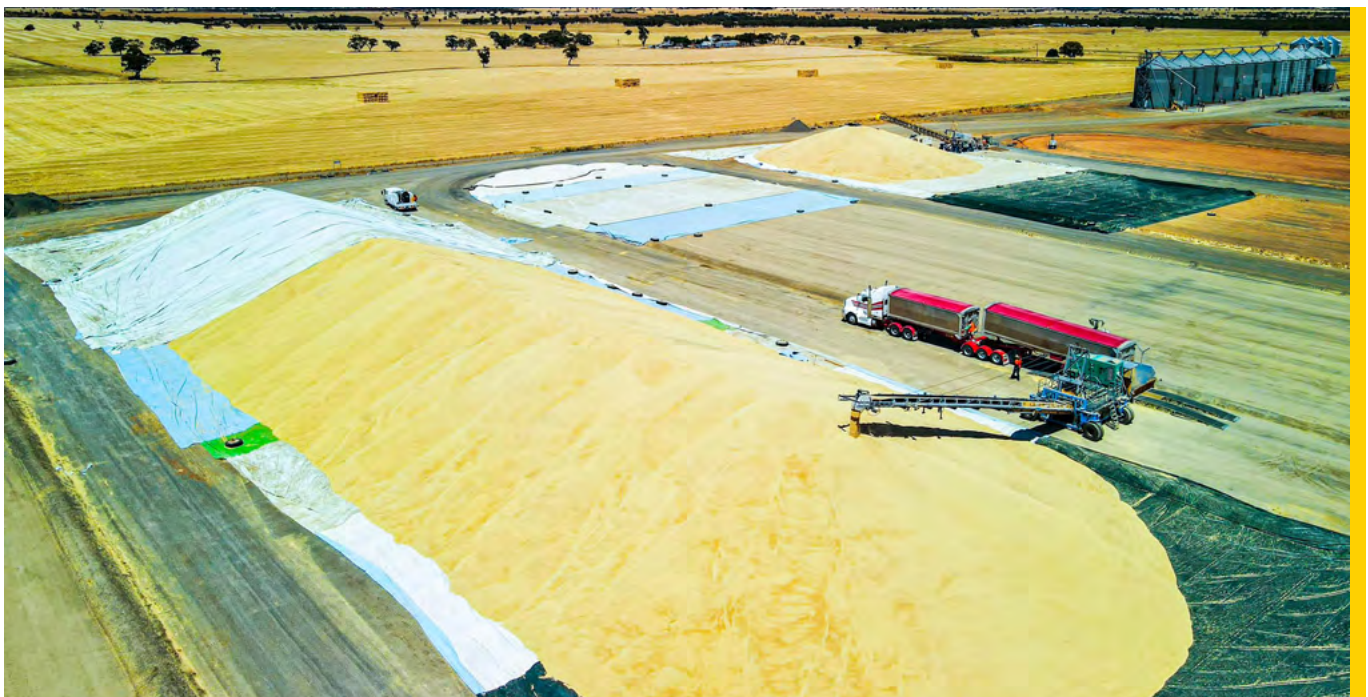
Our regional receival sites along Australia's east coast draw grains and oilseeds from local farms for storage. Both domestic and export markets are serviced from these holdings.
