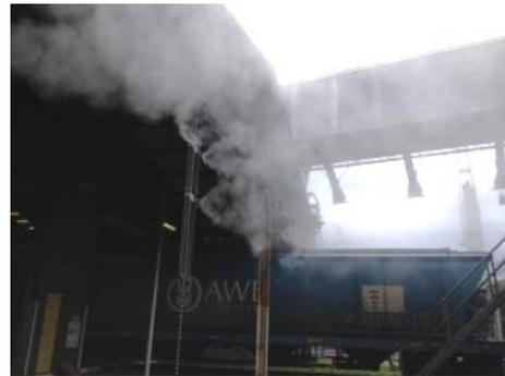
Figure 5 - Rail receival shed water spray
