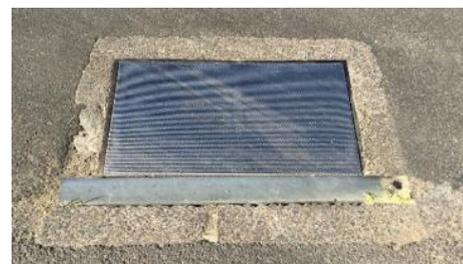
Figure 6 - Stormwater drain equipped with sediment mesh
