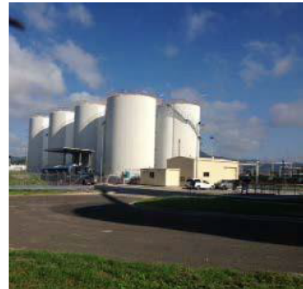
Figure 3. Bulk Liquid Storage Facility
