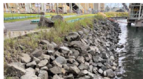
Figure 10. Sediment fences installed along the foreshore
