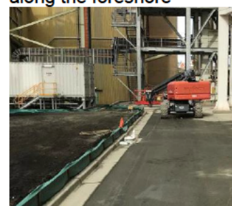
Figure 11. Sediment fences installed along perimeter of affected area by pollution incident
