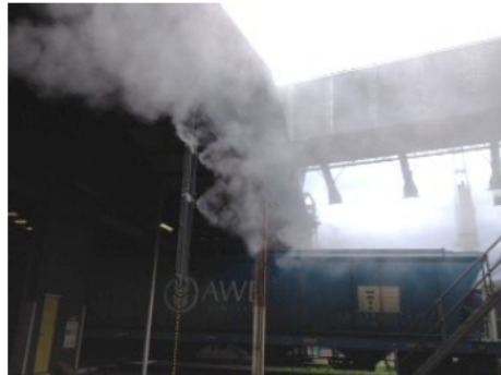
Figure 5 - Rail receipt shed water spray
